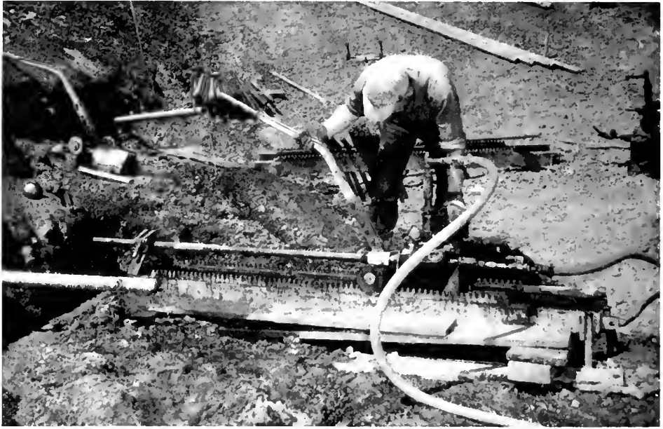
Hydrauger drill in operation
